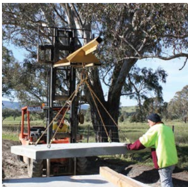
Loading concrete decks
