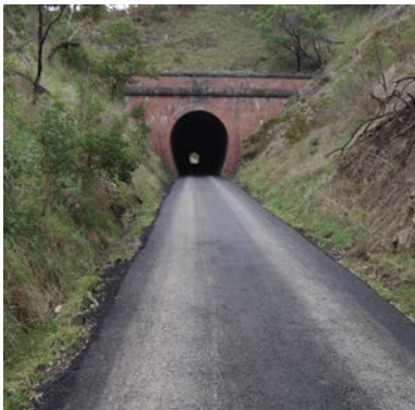
Cheviot Tunnel after track sealing
