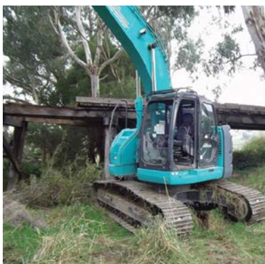
Removing bridge deck timbers
