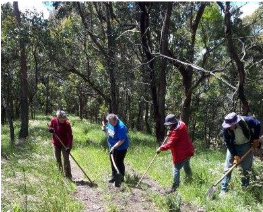
Clearing the former railway alignment for the new trail. Photo: Lindsay Clay
