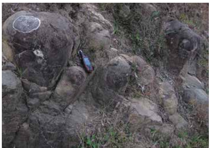
Pt. 13. Spheroidal weathering in thick sandstone of the Esk Formation in the cutting north of Yimbun Tunnel.
